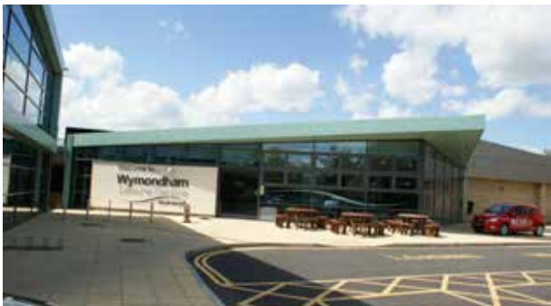
Wymondham Leisure Centre GMV5 Heat Recovery UK
